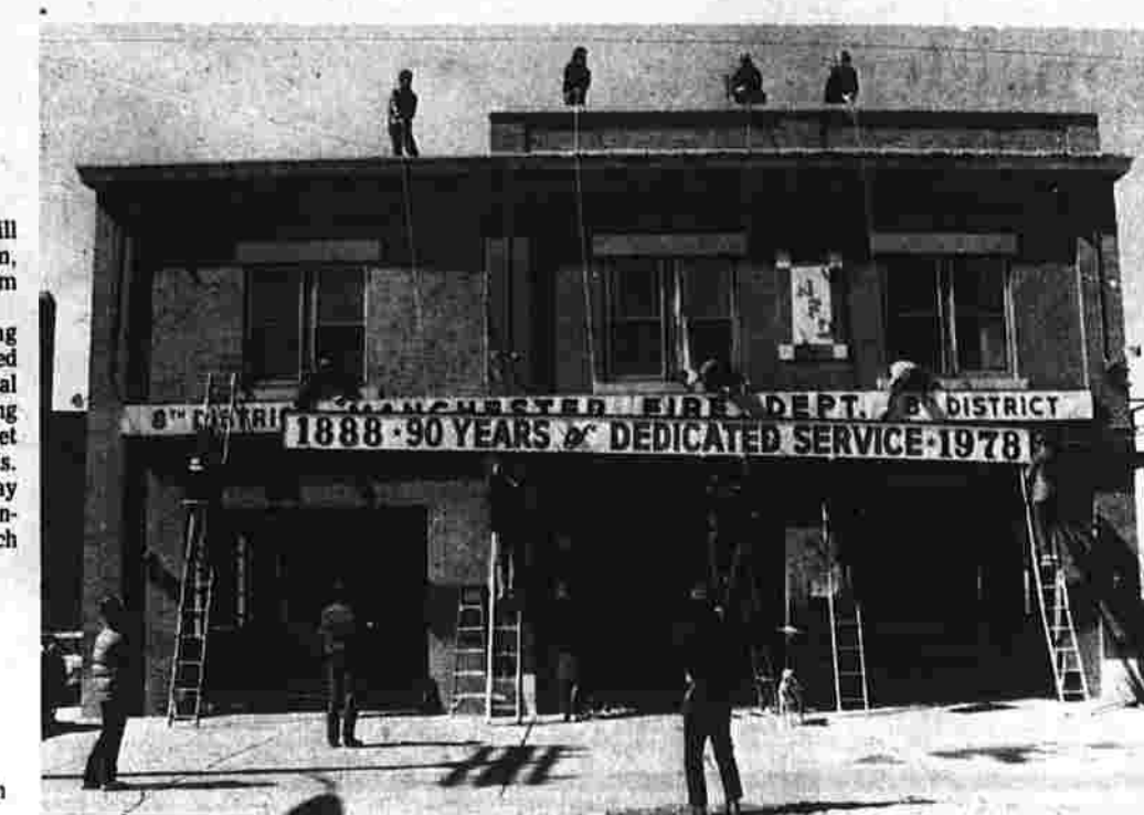
Fire fighters from the Eighth District Fire Department raise a sign to the front of the fire station at Hilliard and Main streets. This year the department is celebrating its 90th birthday. (Photo by Emmet Gemme)
